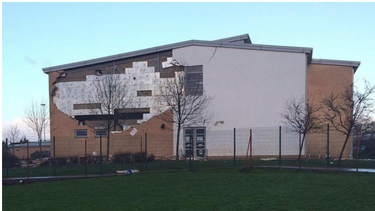
The south gable of Oxfangs School in Edinburgh after the January 2016 collapse. Picture: STV
